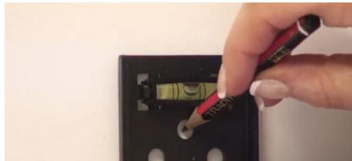
Using the spirit level, mark the wall mount screw positions. Check our how-to guide about getting the perfect height for more guidance.
