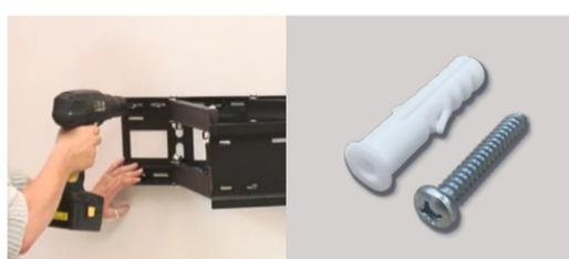
For solid walls, use the electric drill to drill the required 10mm diameter holes. The required depth is included in the instruction manual. Use the included wall screws and plugs to secure the mount to the wall.
