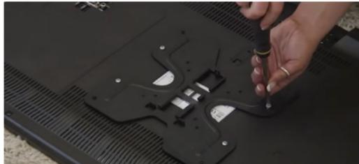
Attach the TV parts of the mount to the TV, so you can check the compatibility before any holes have been drilled in the wall.
